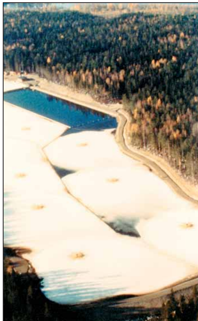
Typical wastewater treatment lagoon at a pulp and paper mill.
