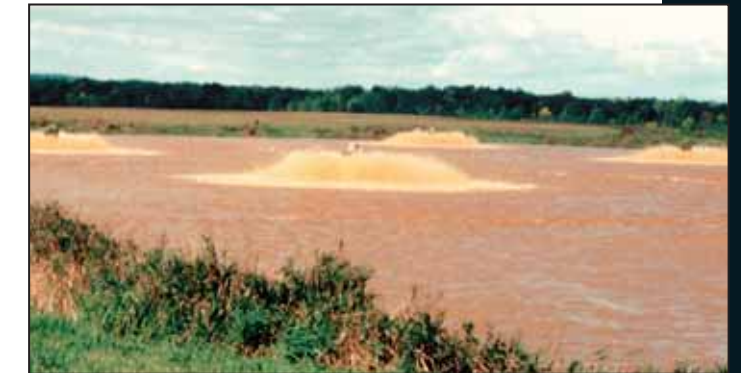
Aqua-Jet® aerators successfully treat the wastewater at a food processing plant.
