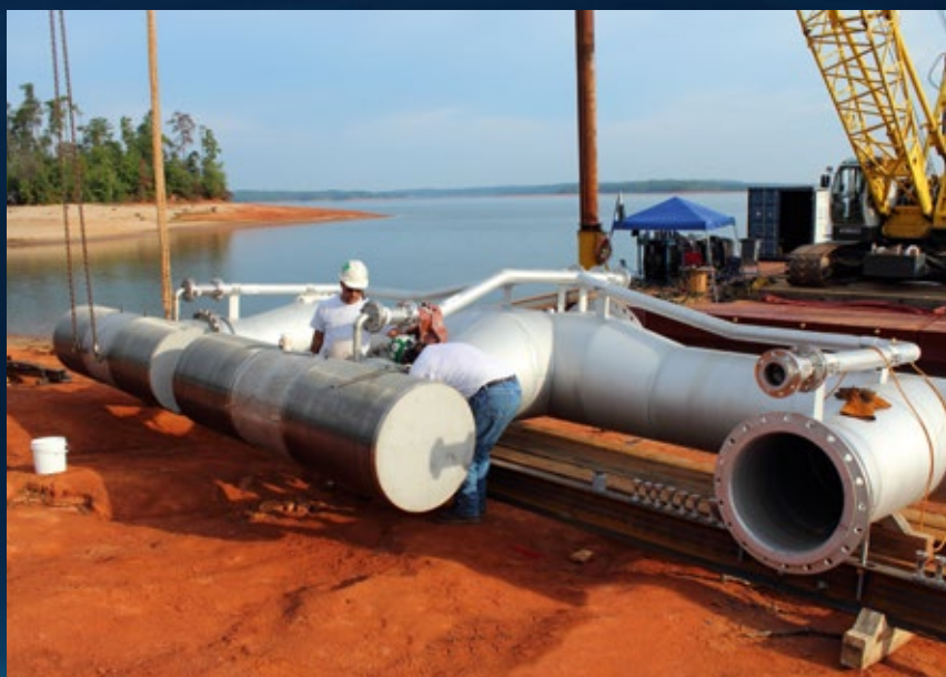
◀ JOHNSON SCREENS® Passive Intake Installation: Drinking Water Plant, in South Carolina, USA
